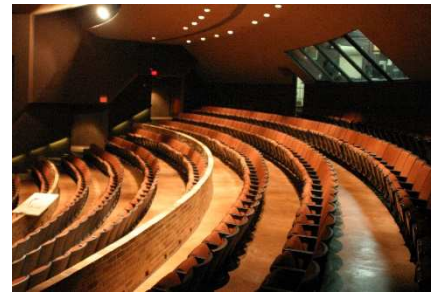
Fire sprinklers in Fain Auditorium
