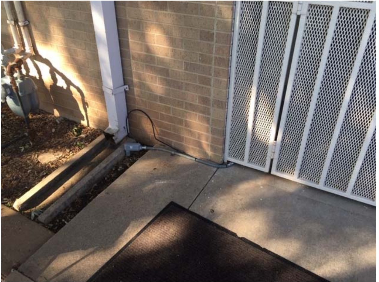
IMG_9804: Existing conduit entrance from ground into caged electrical area.
